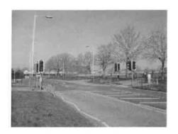
Toucan crossing (including high friction surfacing on approaches) typically costs between £25,000 - £35,000.
