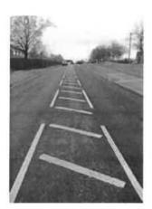
White lining costs up to £1 per metre. Hatching as shown above costs approximately £10 per metre squared. Removal of white lines costs between £12 and £36 per metre depending on the method required. Road studs cost around £15 each.
