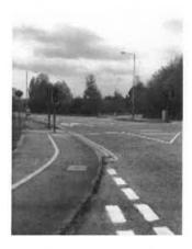
A typical pedestrian refuge, including electrical works and all other associated works, costs between £5,000-£7,000. Refuges allow pedestrians to cross one stream of traffic at a time. They are useful where the concentration and number of pedestrians is fairly low. By narrowing the road, they reduce speeds, but the road needs to be wide enough to allow for a suitable refuge and the safe passage of vehicles and cycles.
