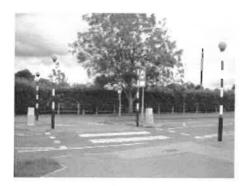
Puffin crossing (including high friction surfacing on approaches if required) typically costs between £25,000-£35,000.
