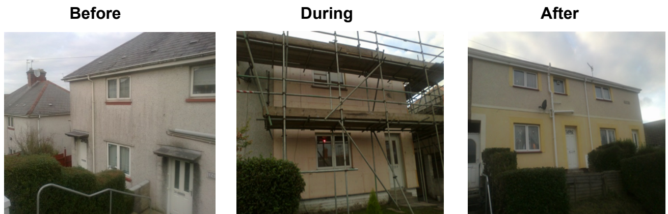
Figure 3 – Typical Enveloping Scheme 1
